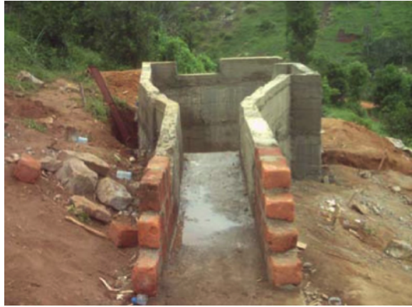
Figure 23 Forebay Tank
